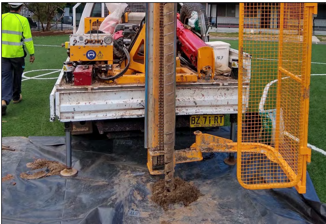
Photo 4 – Soil cuttings retrieved from drilling of BH2
