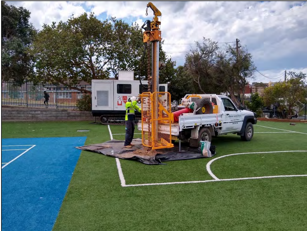
Photo 2 – Drilling in the location of BH3 and performing CPT4
